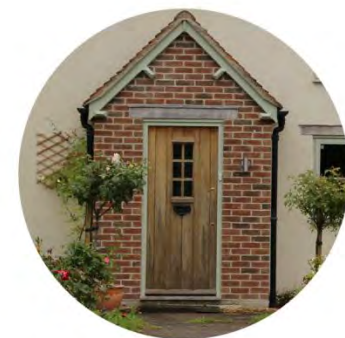
RED BRICK/TIMBER PORCH
